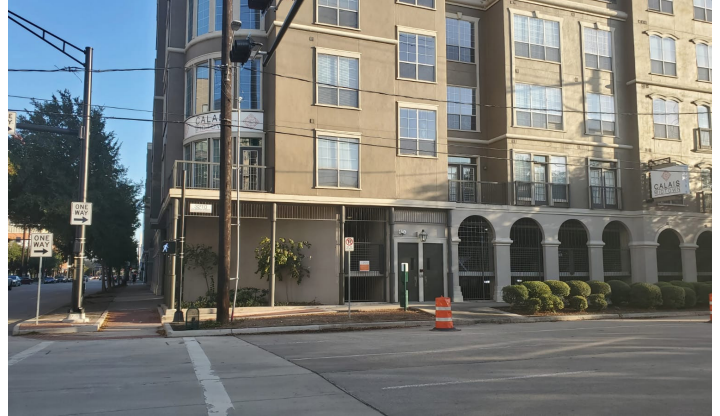
Developer Using Mandated "Active Space" For Parking
